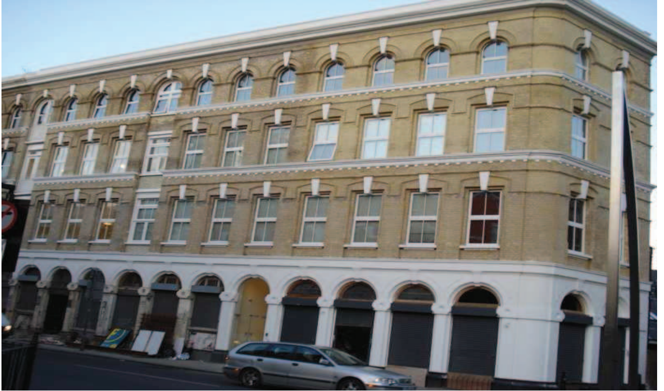
44/48 Commercial Street, LONDON, E1 6LT. We have done the interior design of this project. We were also the structural engineer for renovation of this beautiful building. Client: Dr. Nanda, Nanda Group Ltd
